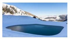
beginning of the season but from the start of this new season, snow can be produced with far greater reliability. Water storage has been increased by a whopping 80% from 170,000 to 306,000 cubic metres and, at the same time, the high pressure pumping capacity has been upped by a third, from 600 to 900 litres / second. At the right temperature and humidity, basic snowmaking can now be completed in 72 hours.
